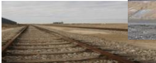
Government-Funded Rail Spur
